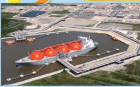
Chorens Energy's Jubba Port terminal, in Somalia, is set to be the first of a new generation of gas processing plants in the region. Phase 1 of terminal construction built 12.7 m 3 of LNG storage in two tanks, each with an LNG capacity of 100,000 m 3 and a maximum combined liquefaction rate of 2.8 mtpa. The layout of any 50 terminal Phase 1 is adding 1.4 mtpa with larger ships set up for 2016-2017. (Photograph: Frank Schreiner/Chorens Energy AG)
